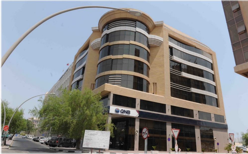
RETAJ OFFICE BUILDING
